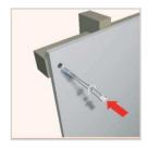
Mark out and drill fixing holes. Insert toggle.
