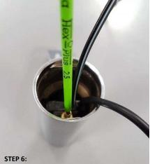
Unscrew (anti-clockwise) brass soap tube fitting with 2.5mm Allen key.
